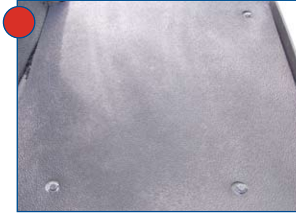
Floor mat unacceptable
