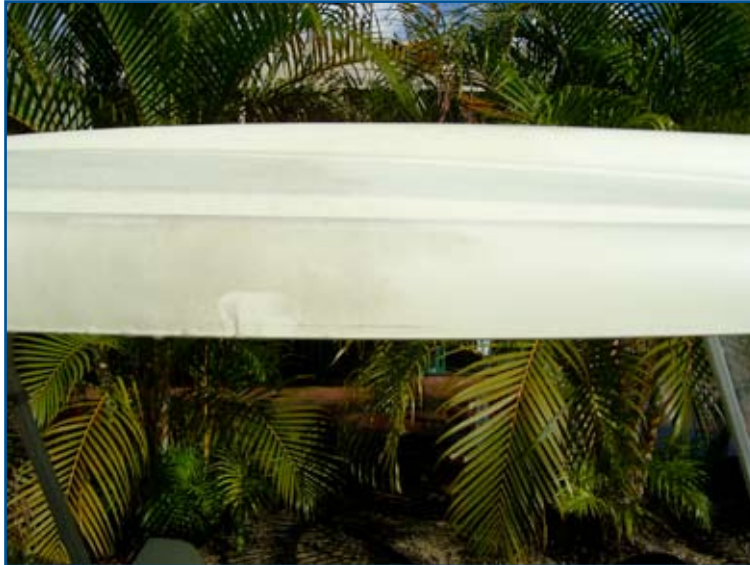
Cleaning line shown
